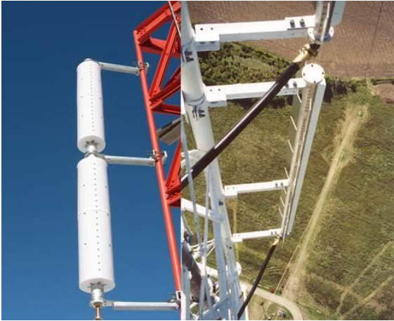
Figure 10: Single section vs. multi-section slotted coaxial antenna designs
