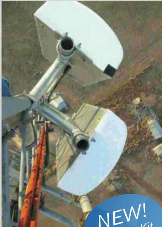
Dielectric's TUA-M Series panel antenna is designed for broadband horizontally polarized operation. The panel is a key building block for antenna system kit. The kit includes flexline jumpers and power dividers, and can be configured to provide antennas with specific azimuth and elevation patterns.
