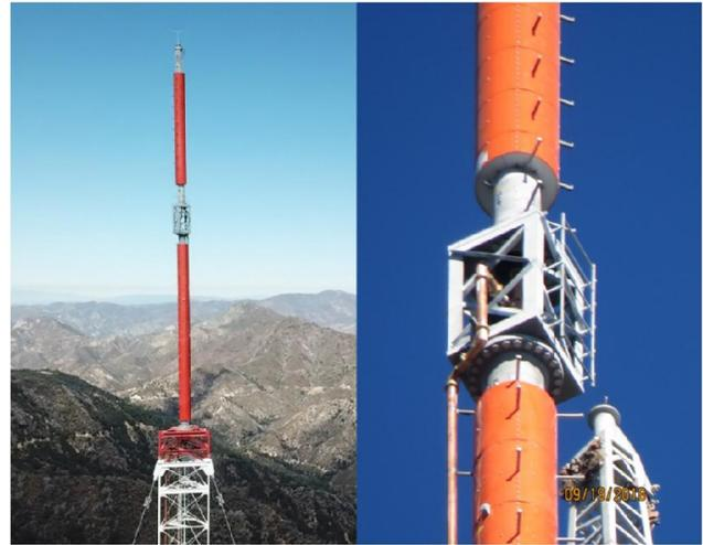
Figure 12: Stacked UHF antenna configuration.
