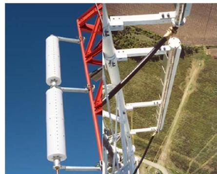
Figure 2: Single section vs. multi-section side mounted slotted coaxial antenna designs
