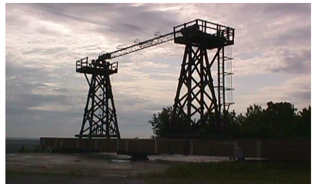
Figure 1: Far field range at Harris Broadcast facility in Palmyra MO.
