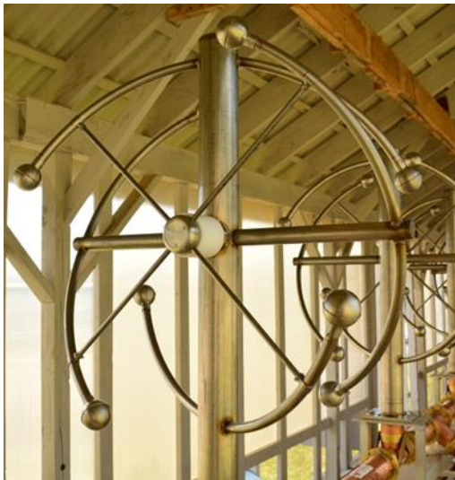
Figure 5: DCRU High power broadband ring style FM broadcast antenna bay.
